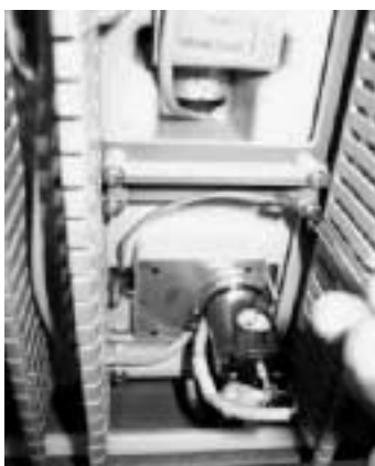
Fig. 126 Unplugging of the electric cable at the Central Computer Board
